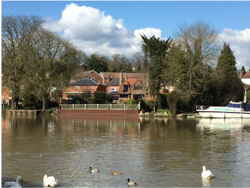
Steel piling of the river bank
