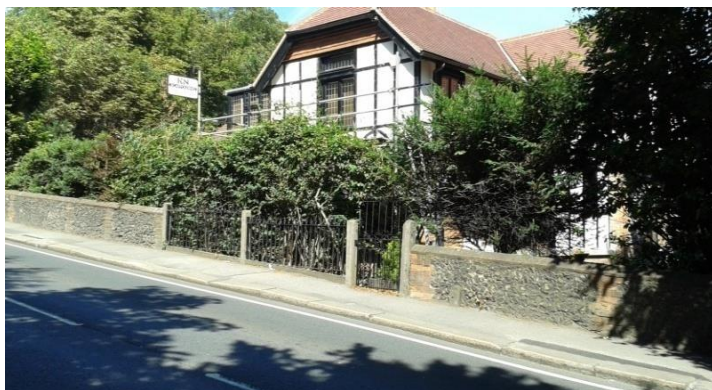
Railings replacing flint walls, St Peters Hill
