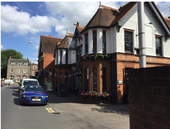
Two 20 th century public houses, the Griffin and the Crown, contribute to the character of the area.
