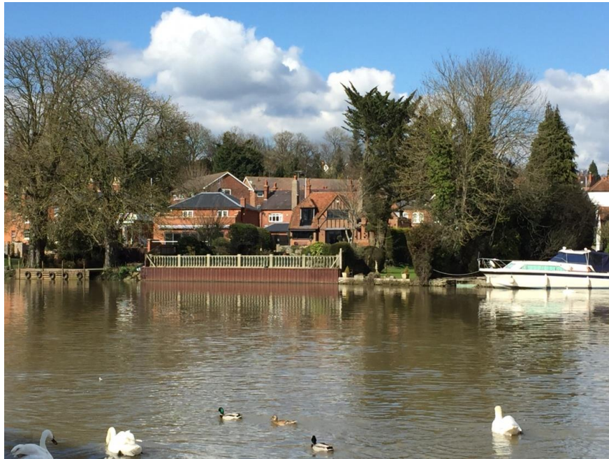
Steel piling of the river bank
