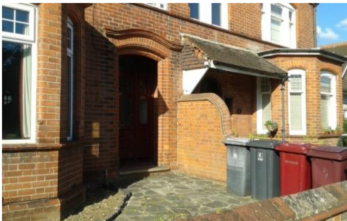
Gravel/paving frontage, removal of greenery, bins in front
