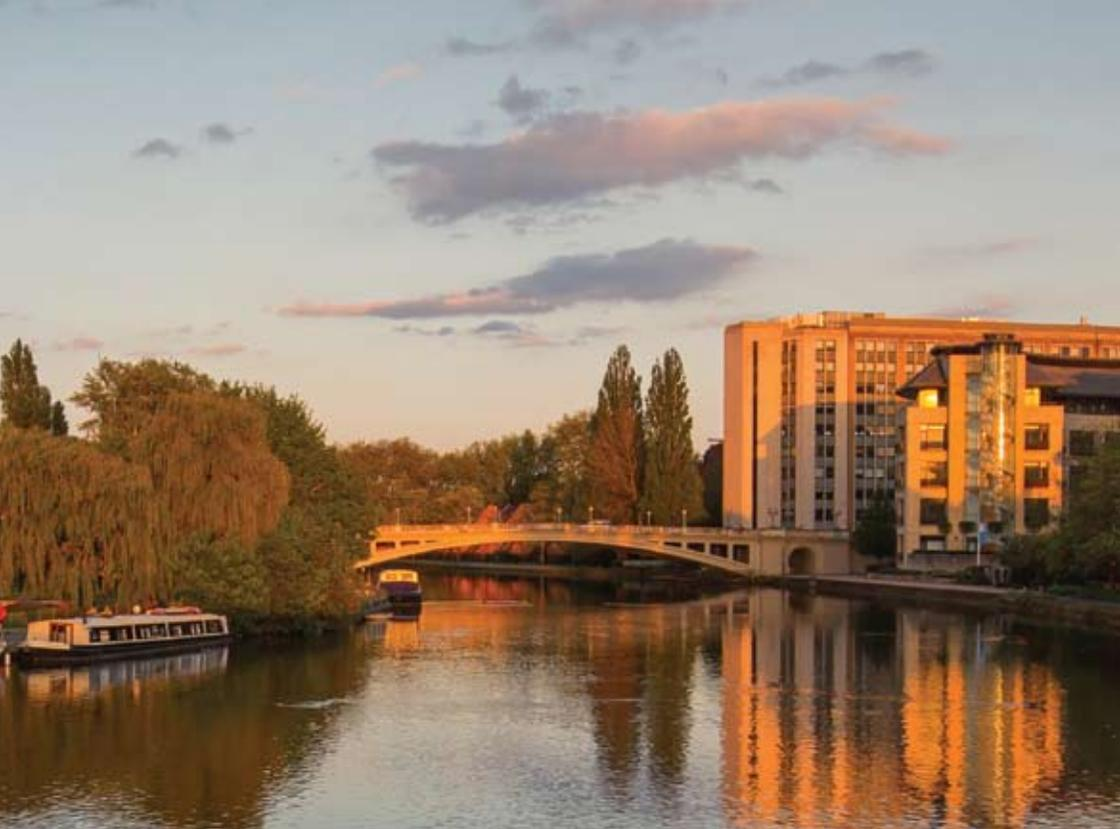
Reading Bridge was opened on 3 October 1923. It is a remarkable example of modern bridge construction in reinforced concrete, simple yet striking in appearance and set off by Portland stone parapets and an elegant line of lamps. Reading Bridge had the longest single span in the UK until 1928. Many other bridges of this period are Grade II or II\* listed.
