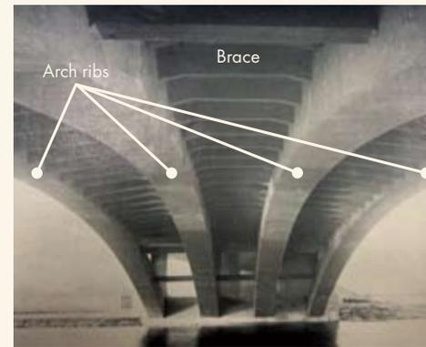
The main structure of the arch is formed by four reinforced concrete ribs 180 ft (55m) long, rising to 18 ft (5.5m) at the centre, linked by braces.
