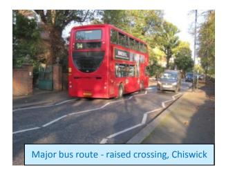
side of the crossing would have a gradient suitable for the passage of buses (typically 1:15 as used for London buses). This would have the effect of slowing traffic and producing a more comfortable crossing for all users, but especially for wheelchair and pushchair users and people with walking difficulties.
