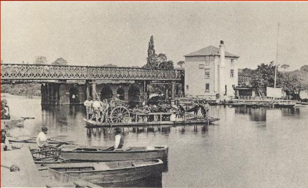
1. REBUILDING CAVERSHAM BRIDGE 1869
