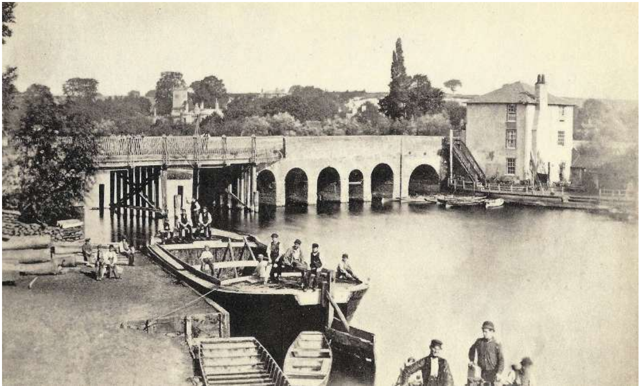
Old postcard showing barge building on the Reading bank, the wooden section on the Reading side, the stone arches on the Oxfordshire side and the Waterman's cottage. Courtesy of CADRA
