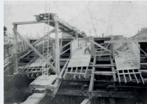
▲ The shuttering for casting the main spans. Image: CADRA
