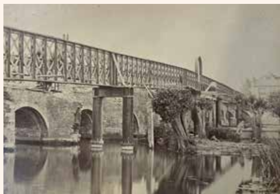
▲ The new iron bridge was initially constructed over the old stone arches, with pillars driven into the riverbed by a screw action, using a capstan. Image: Reading Museum, 191.120.1
