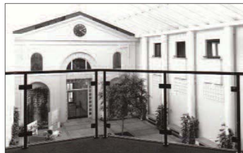
The first modernisation programme in the 1980s saw the refurbishment of the main building
