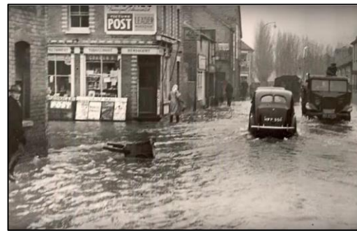
Flooding on George Street in 1947
