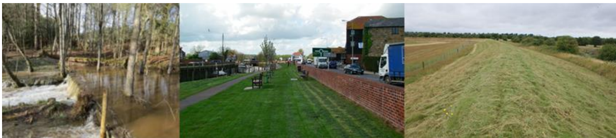
An example of some of the options considered: Natural flood management, flood walls and flood embankments.
