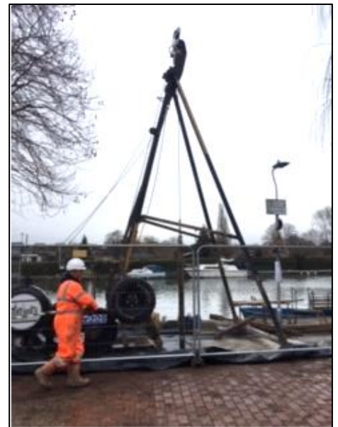
Borehole drilling on the south bank towpath on 18 February 2019.
