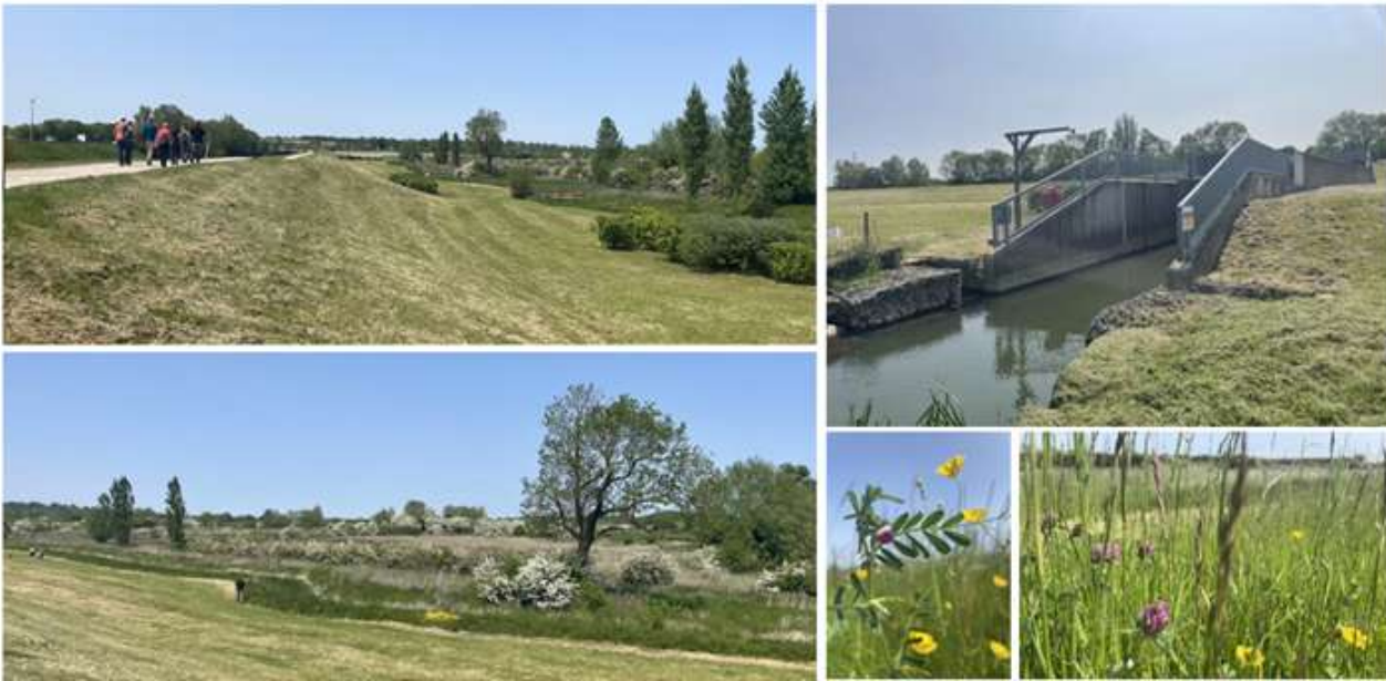
Banbury Flood Storage Area left to right: A sloping embankment made with local materials, a flow control structure, shrubs, trees and long grass within the storage area, close up of wildflowers, common vetch, clover and buttercups.
