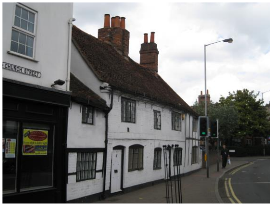
Link to adjacent cottages in Church St. 2011
