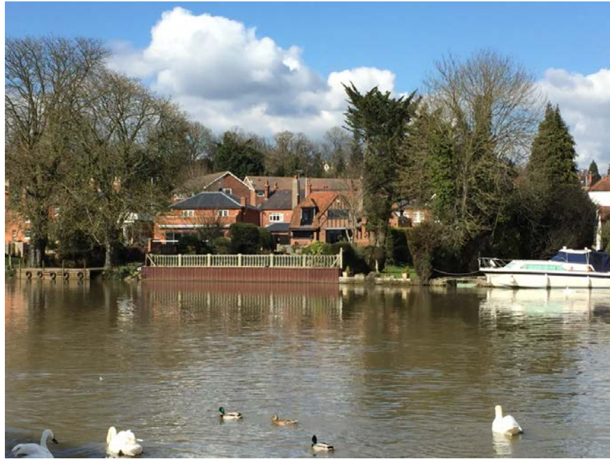
Steel piling of the river bank
