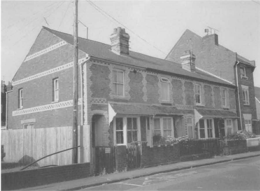
Fig. 7. Terrace houses in Short Street.
