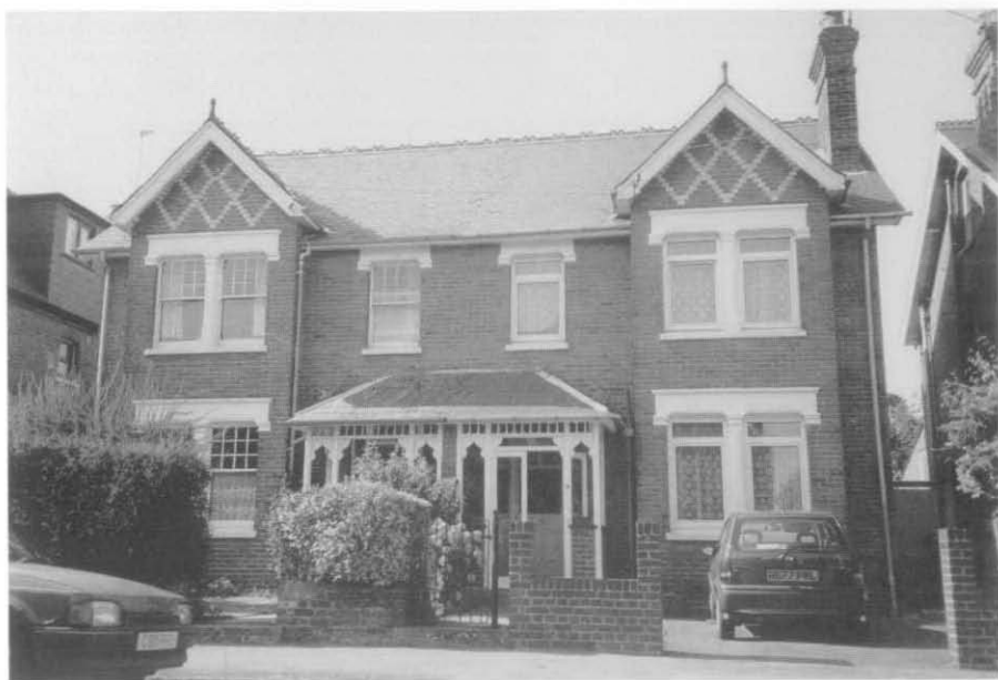
Fig. 18. Semi-detached villas: 9-11 South View Avenue. Red brick with diamond-patterned gables in cream. Architects: W.G. Millar & S. Cox, 1902.
