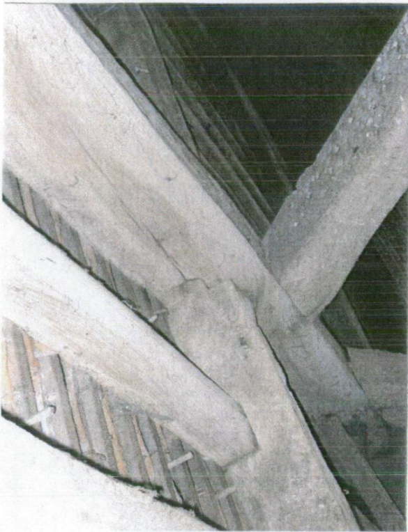
Plate 21 - Lower purlin to principal rafter detail.
