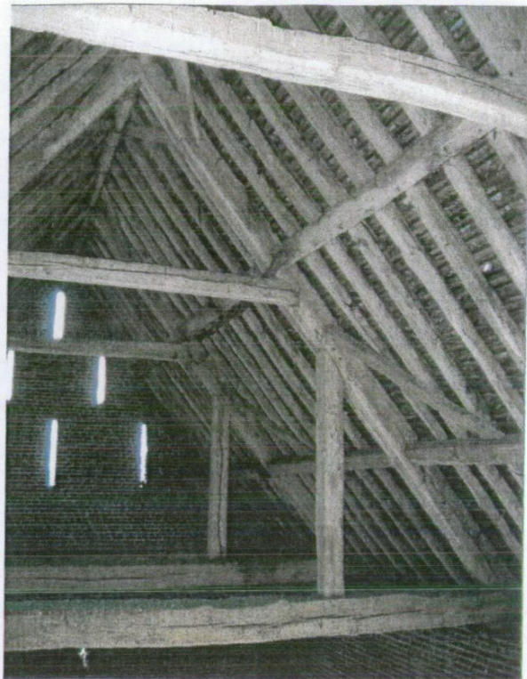
Plate 10 - Detail of last three western bays.
