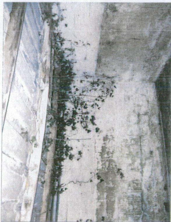
Plate 36 - Internal of southern room in building B.
