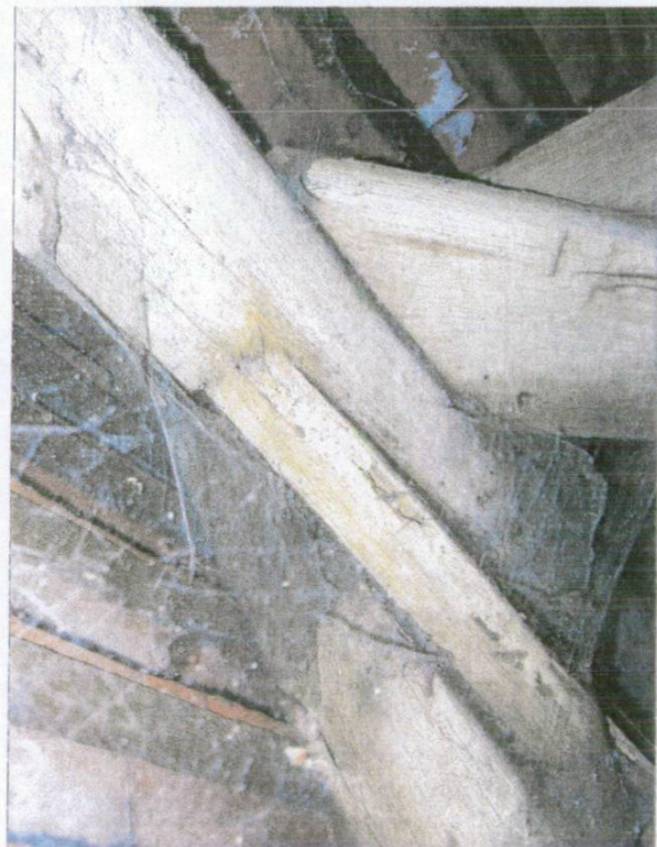
Plate 20 - Brace to ridge detail.
