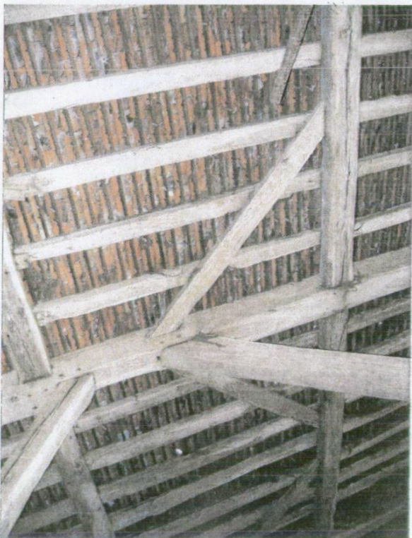
Plate 11 - Detail of principal rafter jointing.
