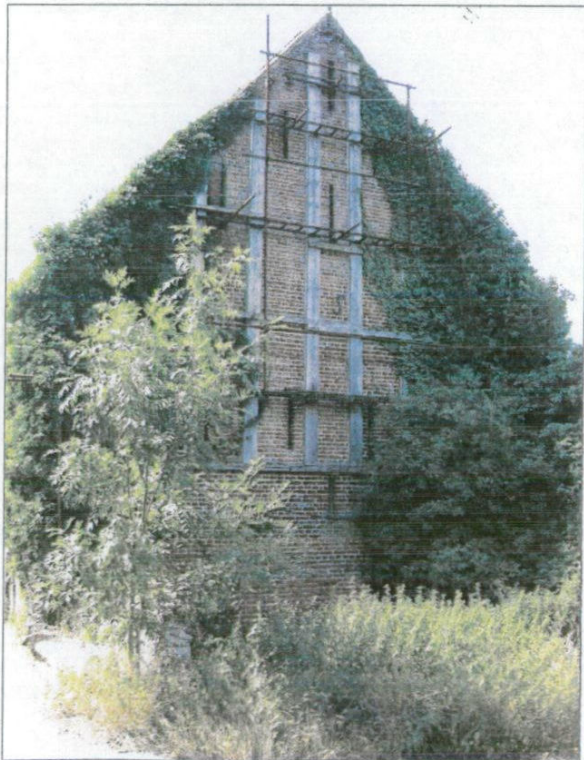
Plate 3 - East elevation of main barn, showing bracing to the brickwork.
