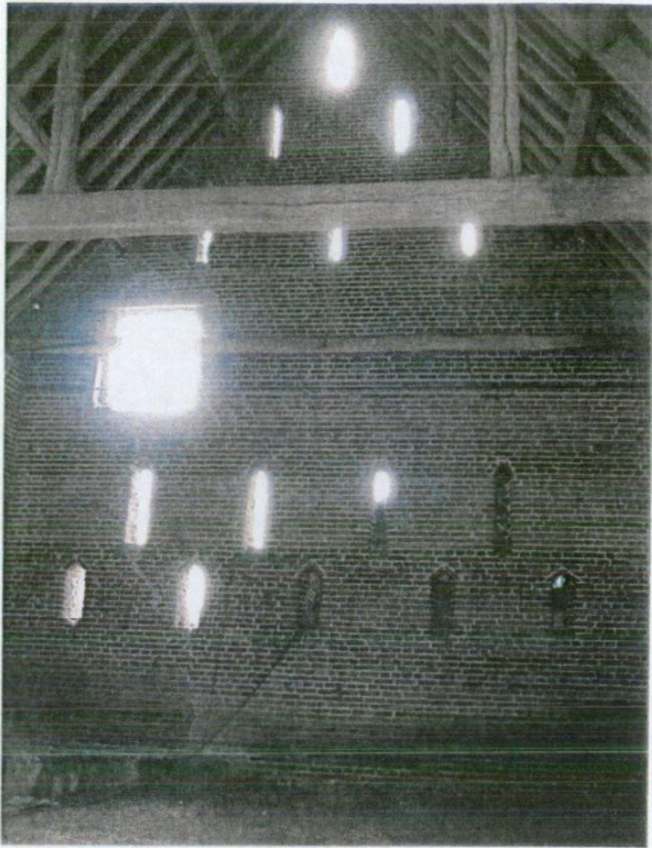
Plate 29 - Overall shot of western internal elevation.
