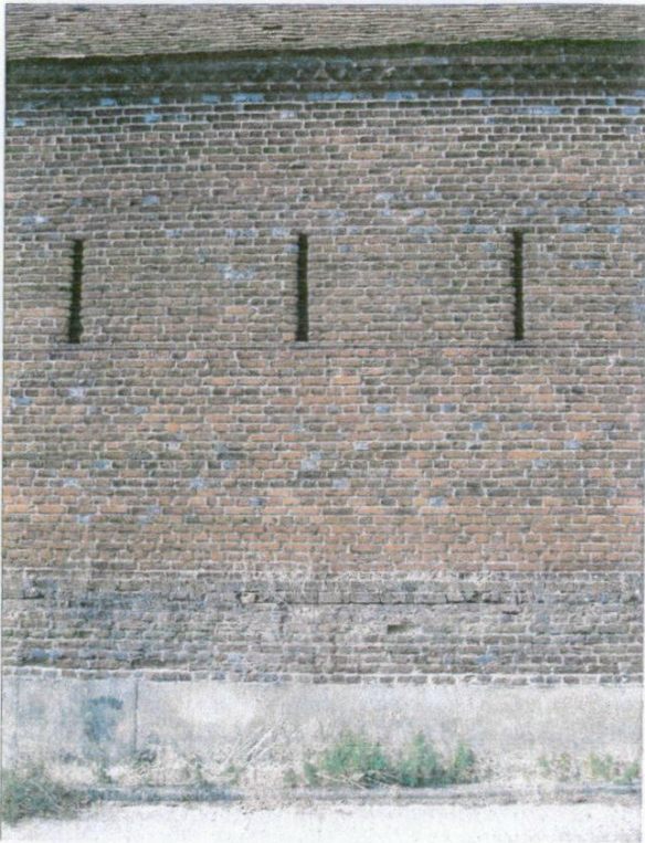
Plate 5 - South elevation of main barn, showing window openings, and concrete underpinning.
